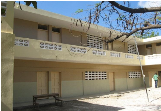
School of La Tremblay, rebuilt and renovated; fully repainted.
