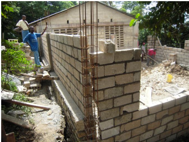
School of Molière, construction work is progressing.
