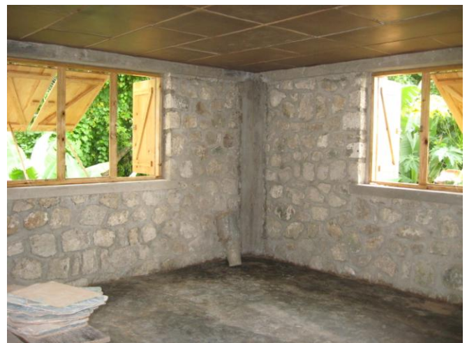
School of Nicolas ,rebuilt; these walls had collapsed on January 12.
