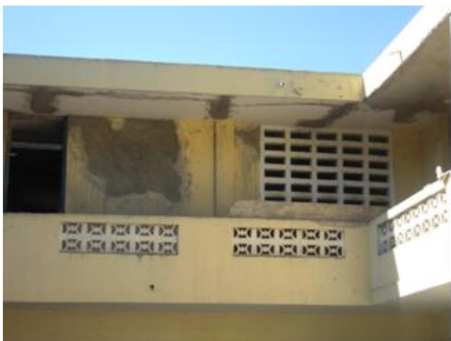
La Tremblay school, construction work is underway.
